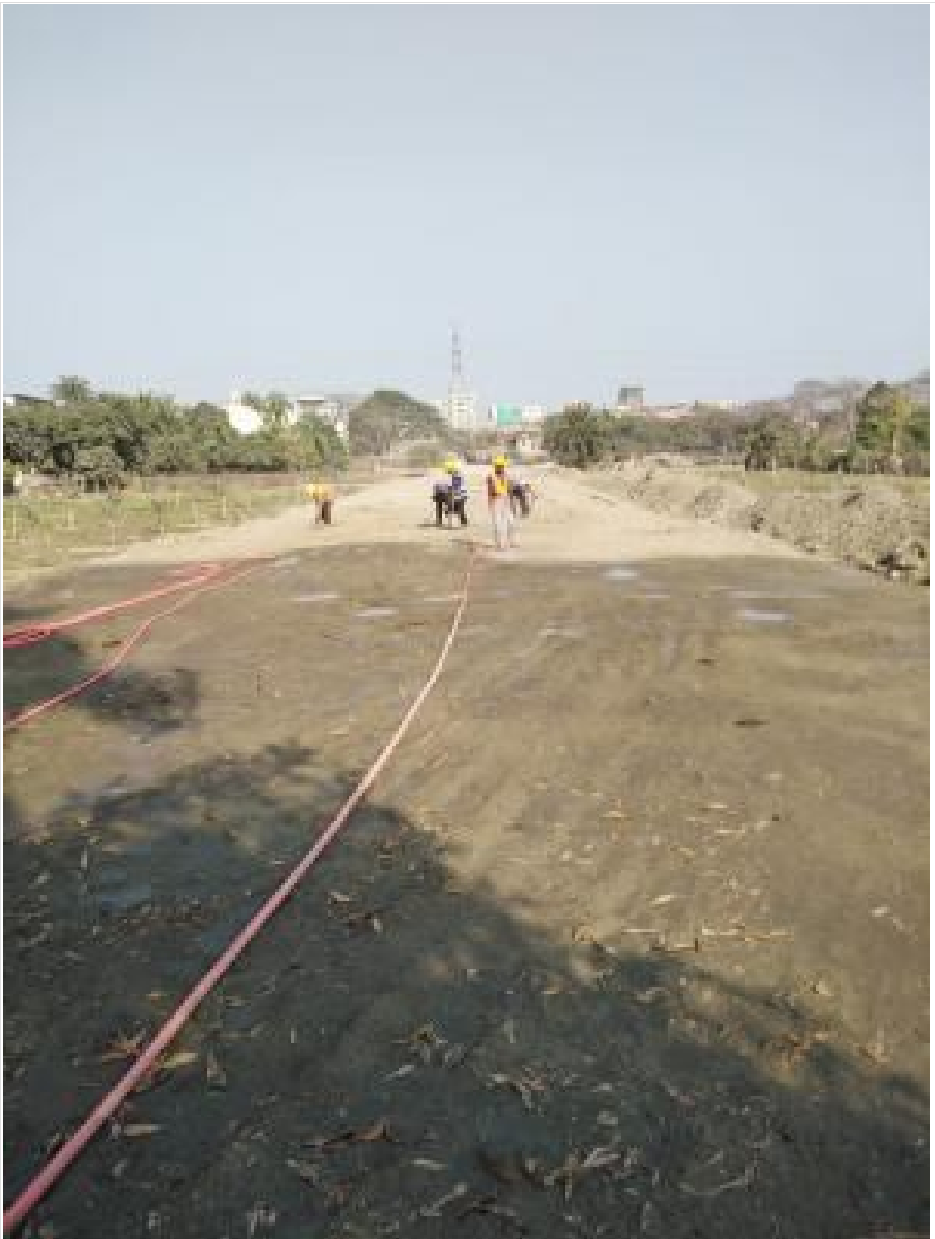
40 ft Road Dressing and Levelling
