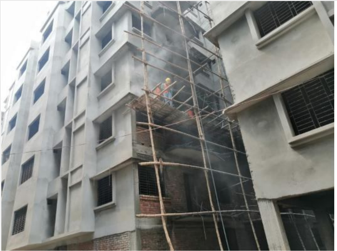
Building Outside Plastering
