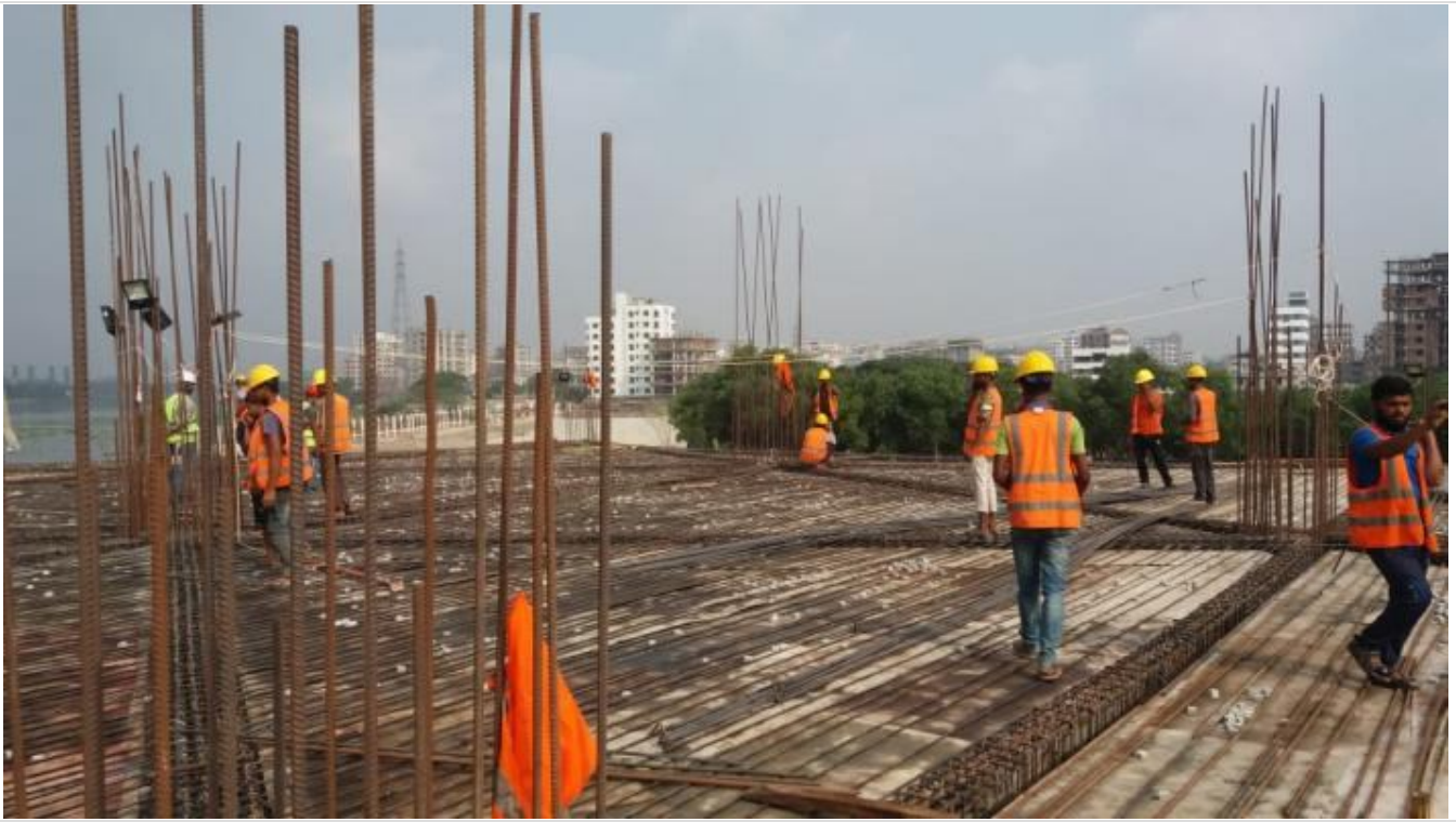
Mosque 1st Floor Slab Re-bar Work
