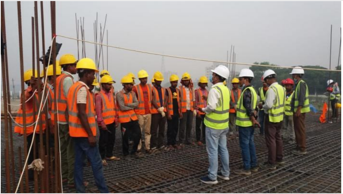
Briefing instruction before Concreting
