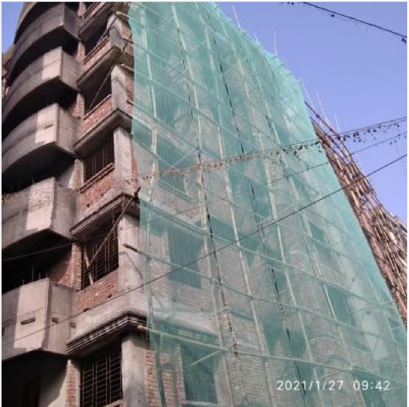
Scaffolding for Outside Plaster-Buildin
