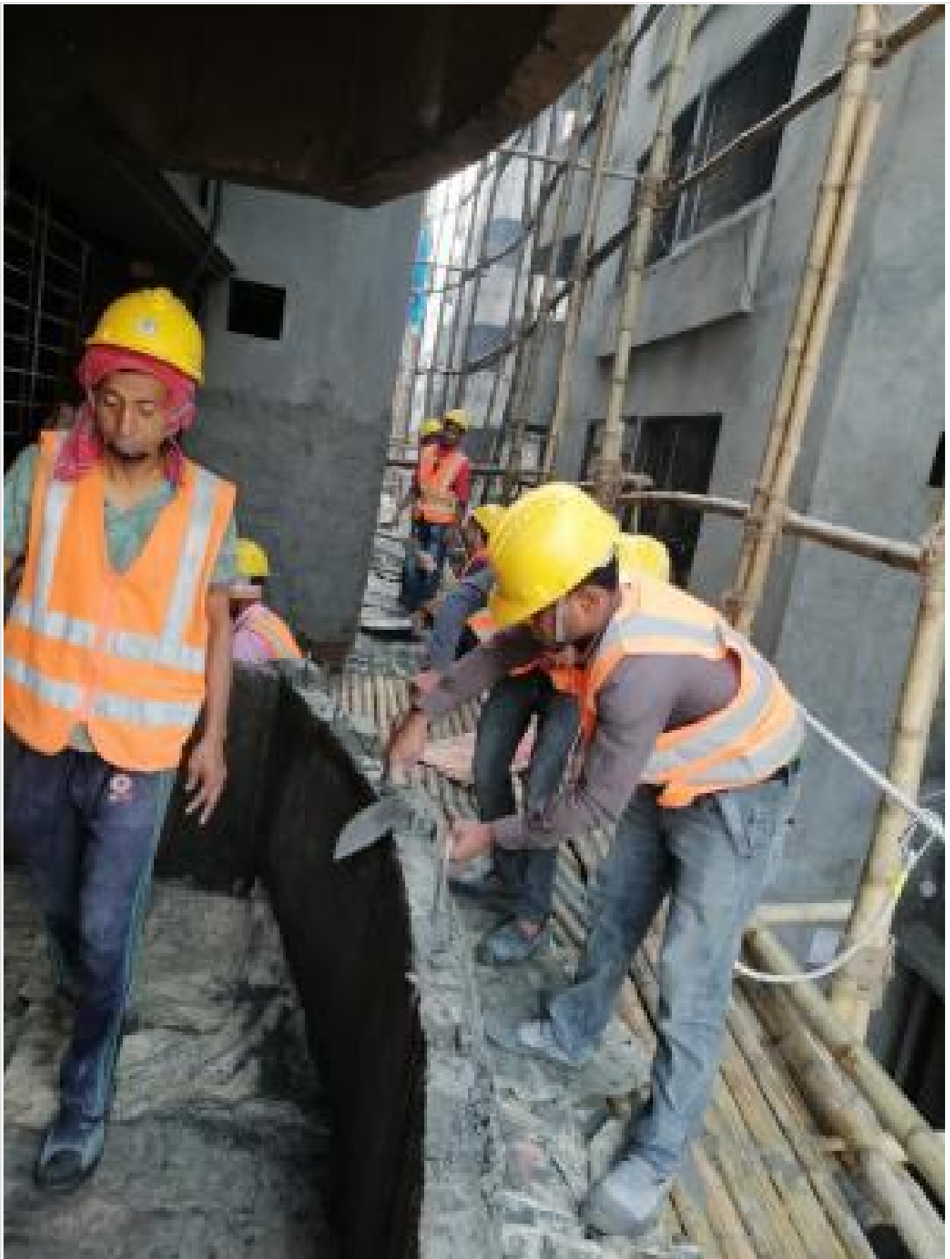
Out-side Plaster Work
