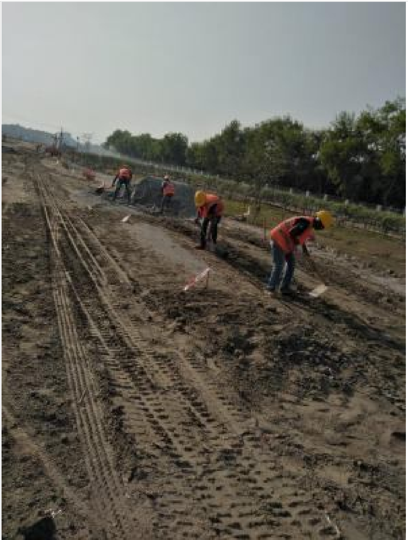
40 ft Road Levelling and dressing
