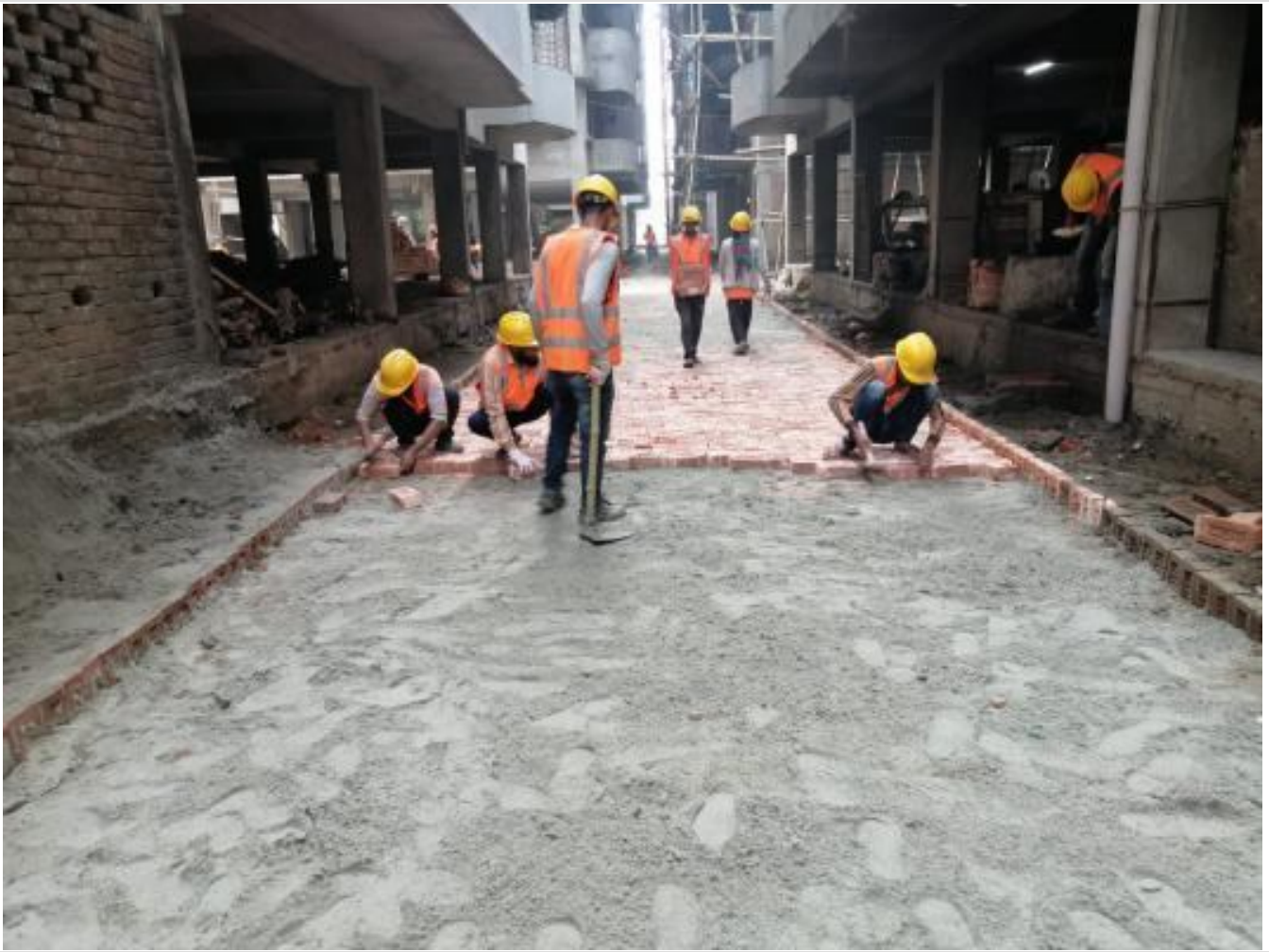
Inner Road CC Work
