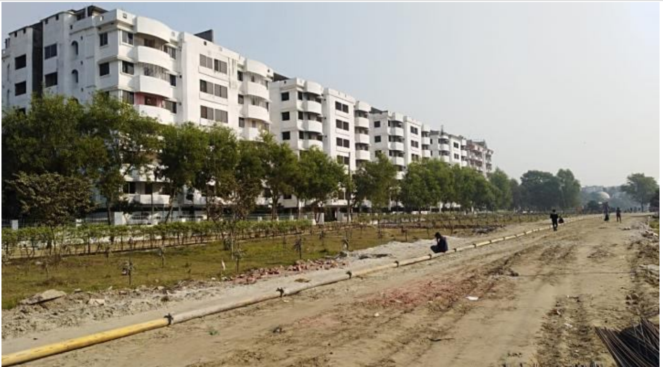
Building Outside Painting
