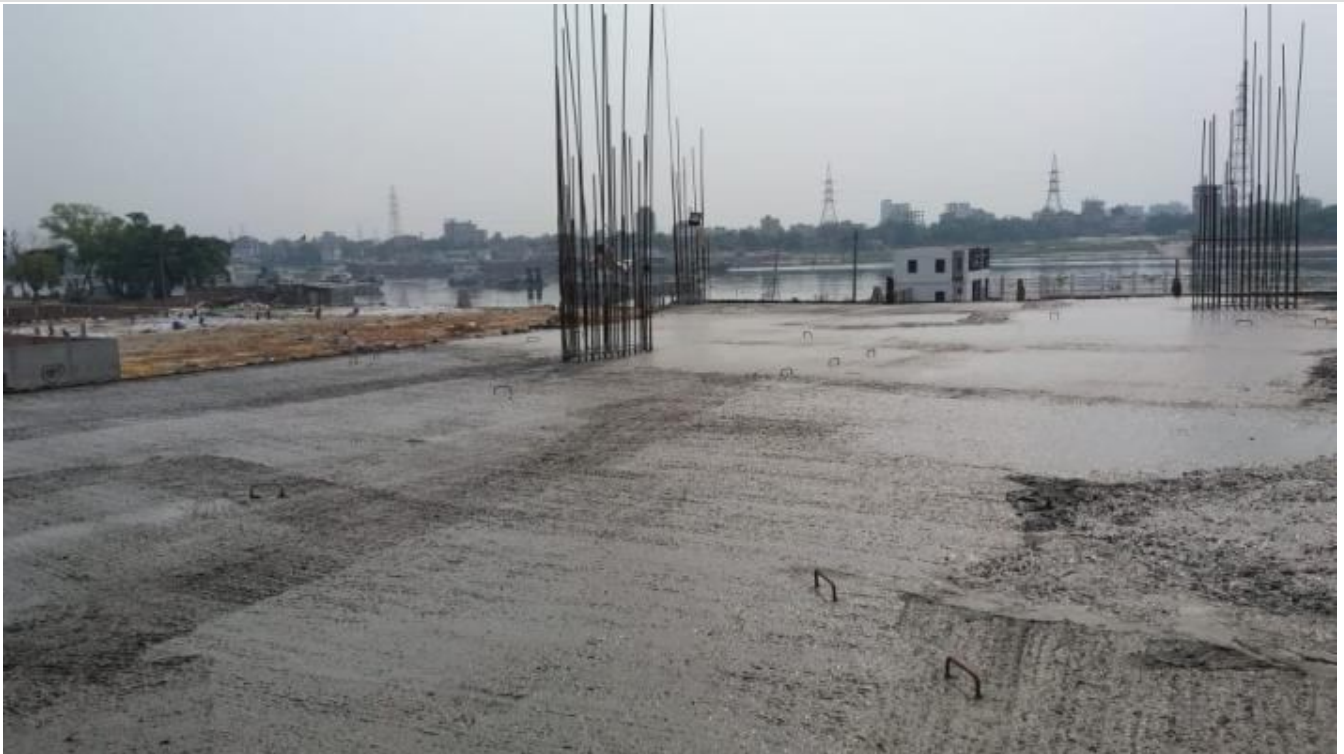
Mosque 1st Floor Slab Concreting
