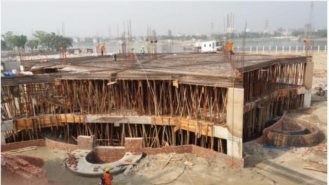
Mosque Building in Construction
