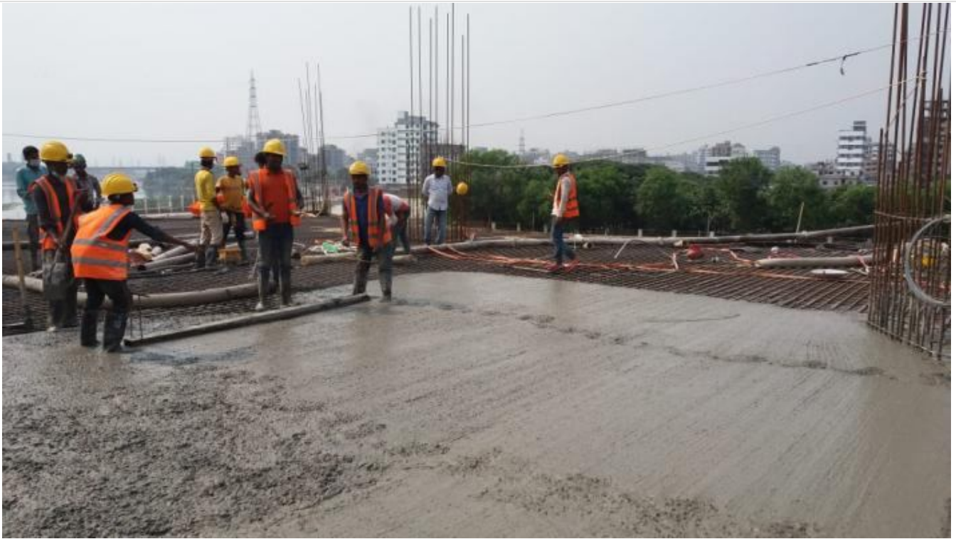
Mosque 1st Floor Slab Concreting
