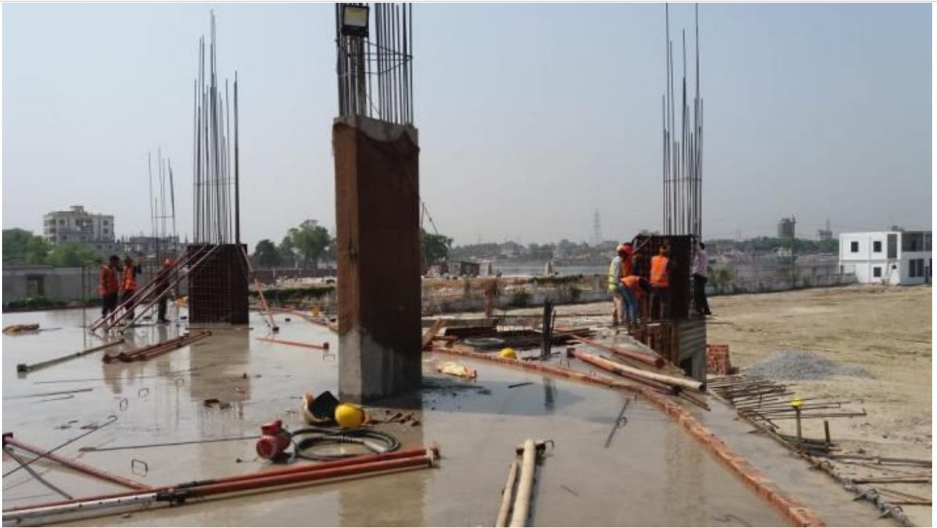
Mosque-GF Column Work
