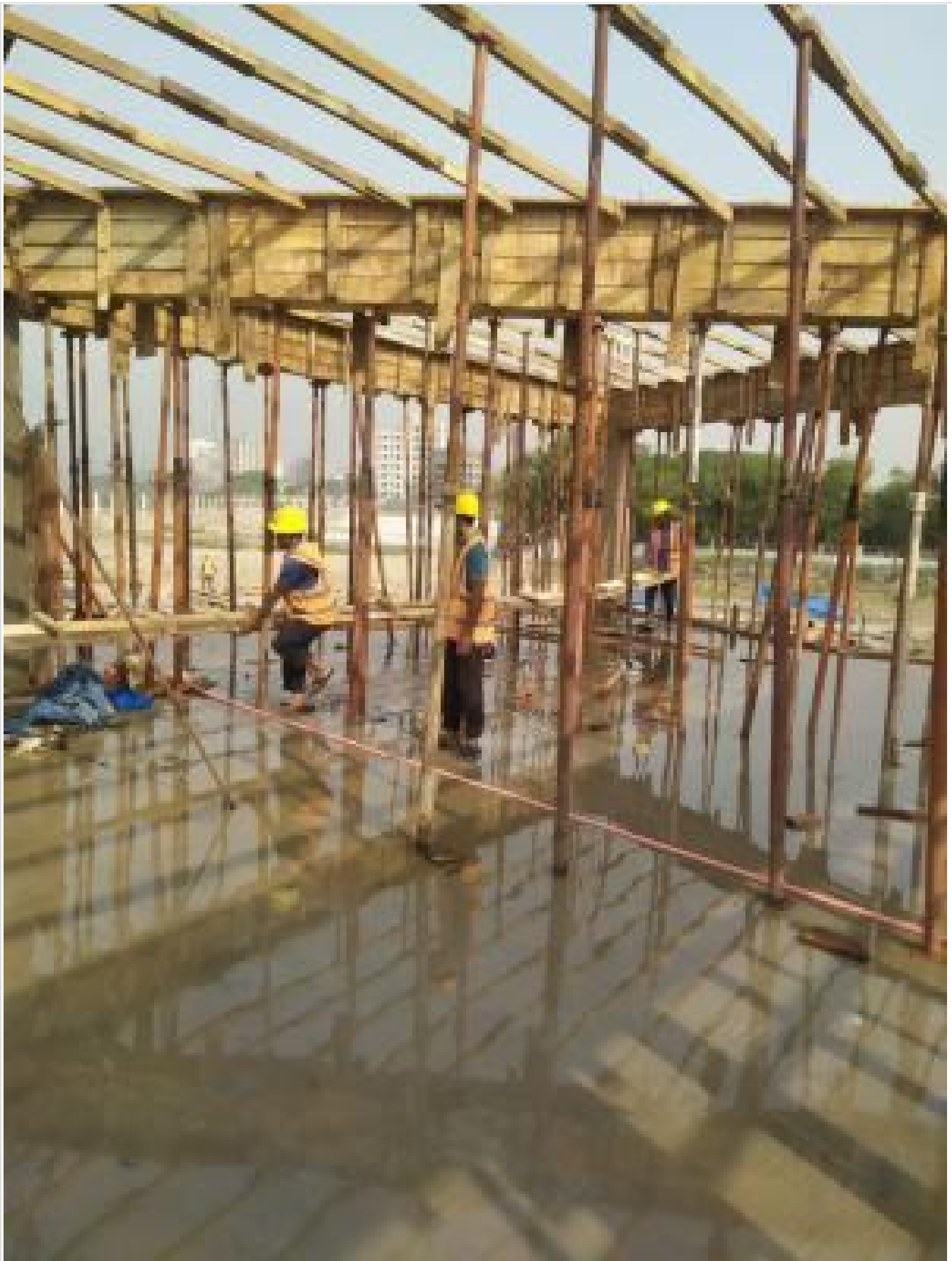
Mosque 1st Floor Slab Shuttering
