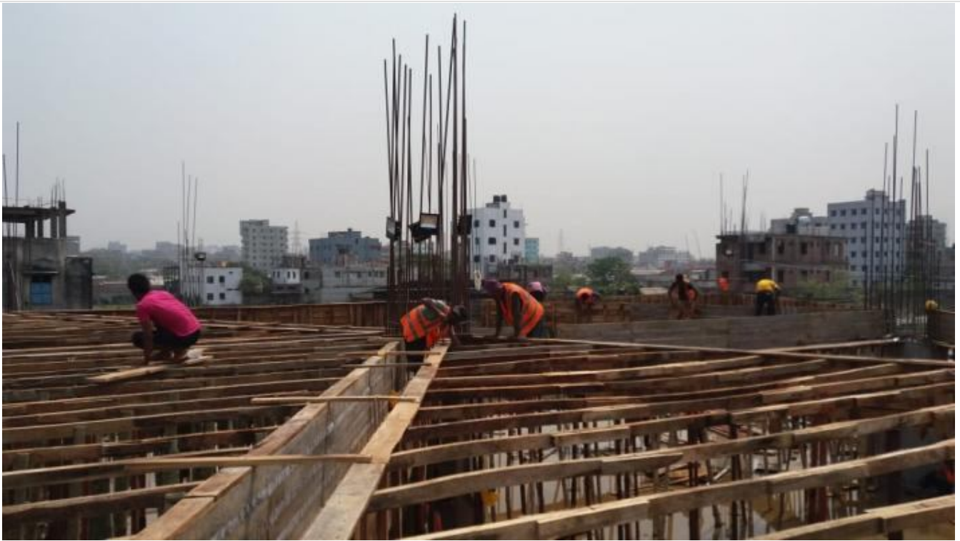
Mosque 1st Floor Slab Shuttering
