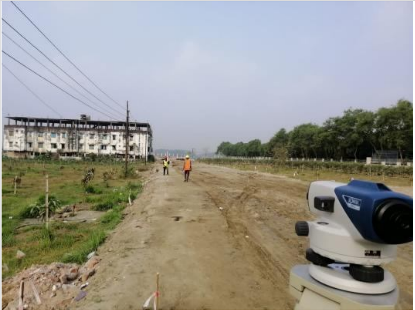
40 ft Road Dressing and Levelling
