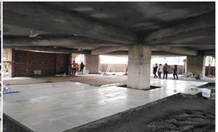
Mosque-Basement Tiles Work
