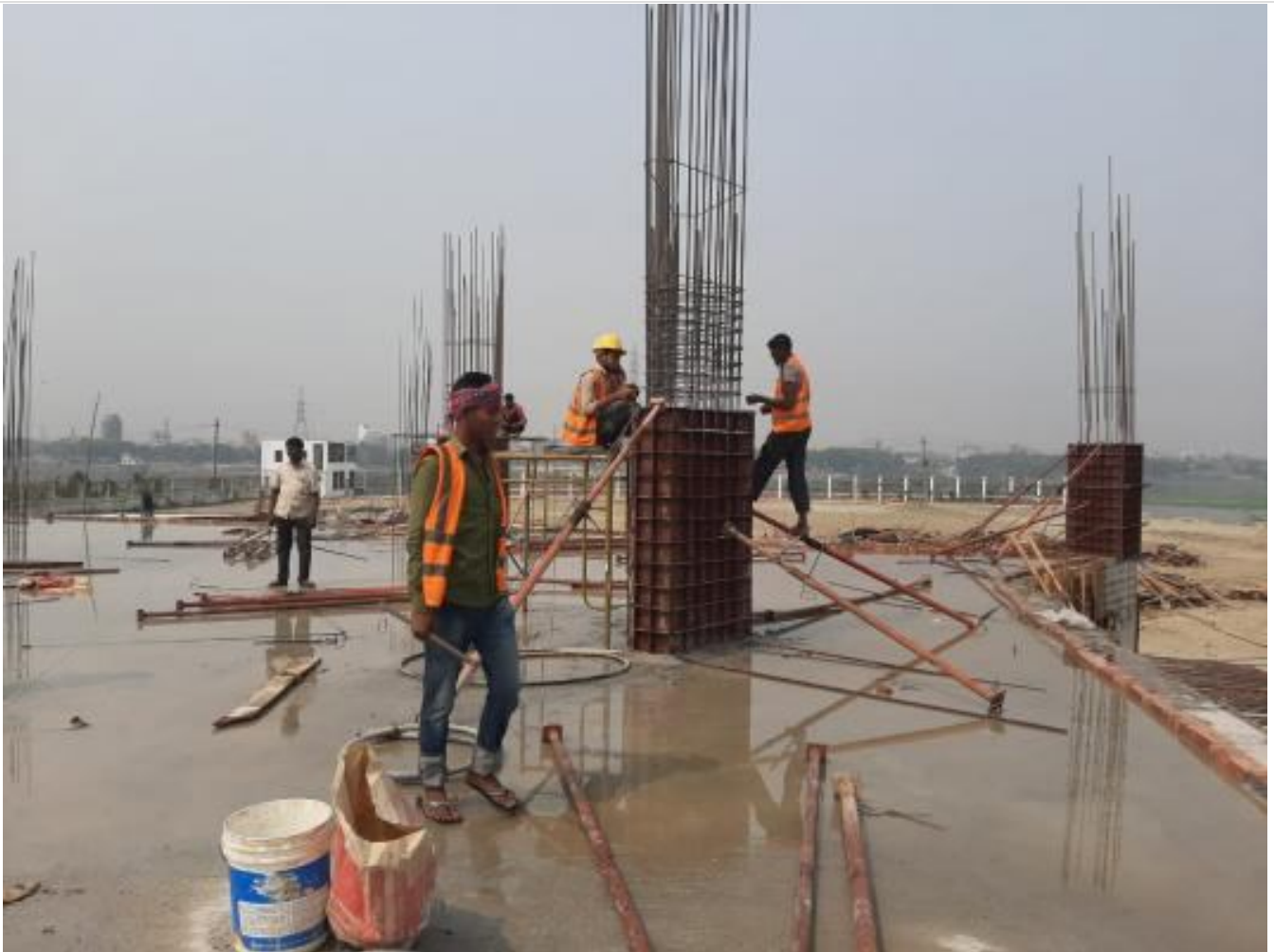
Mosque GF Column 2nd Lift Re-bar Work
