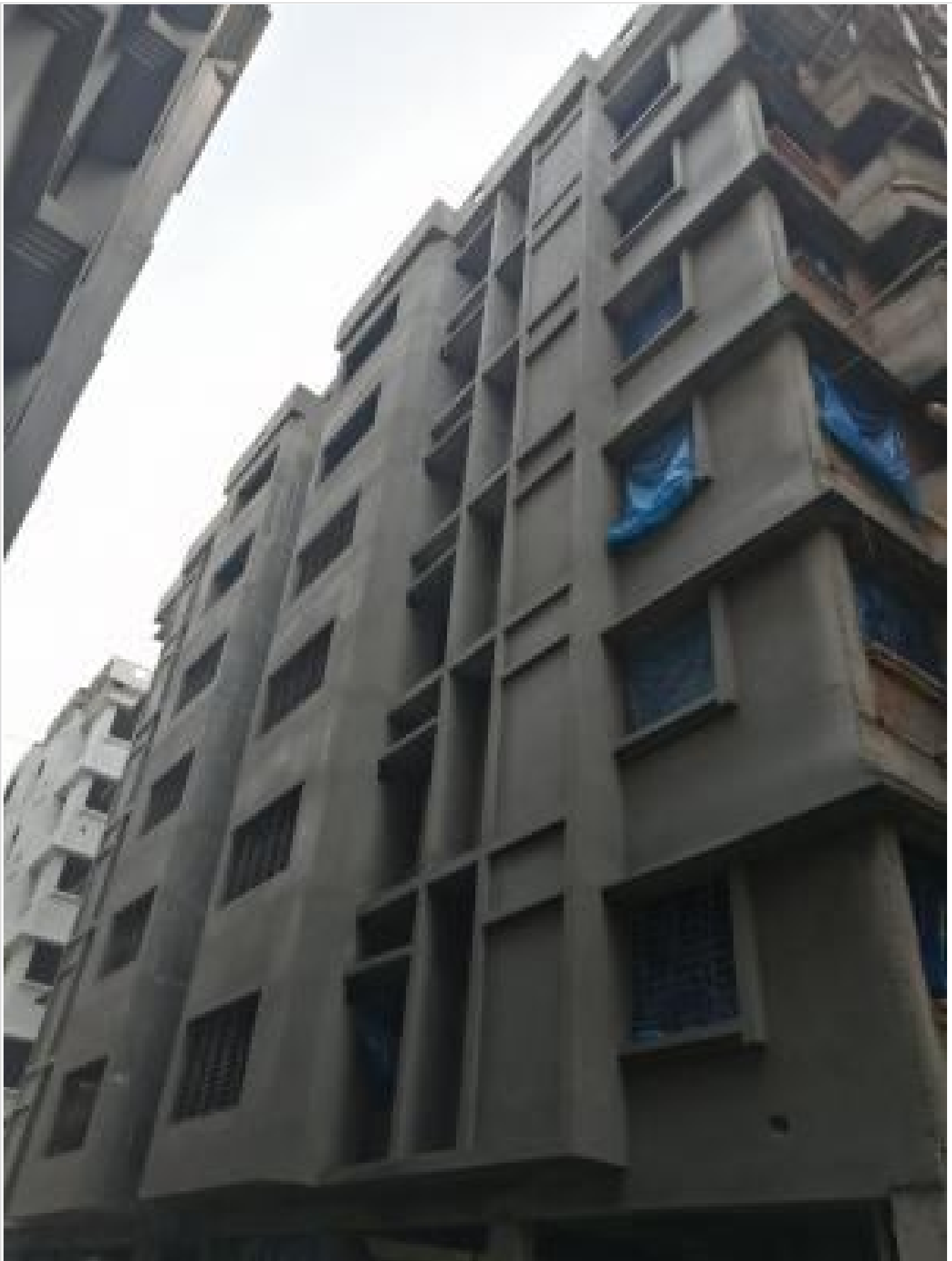
Building-J outside plastering
