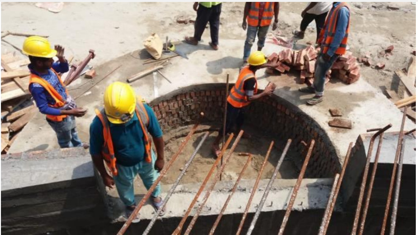
Mosque Ground Floor Stair Concreting
