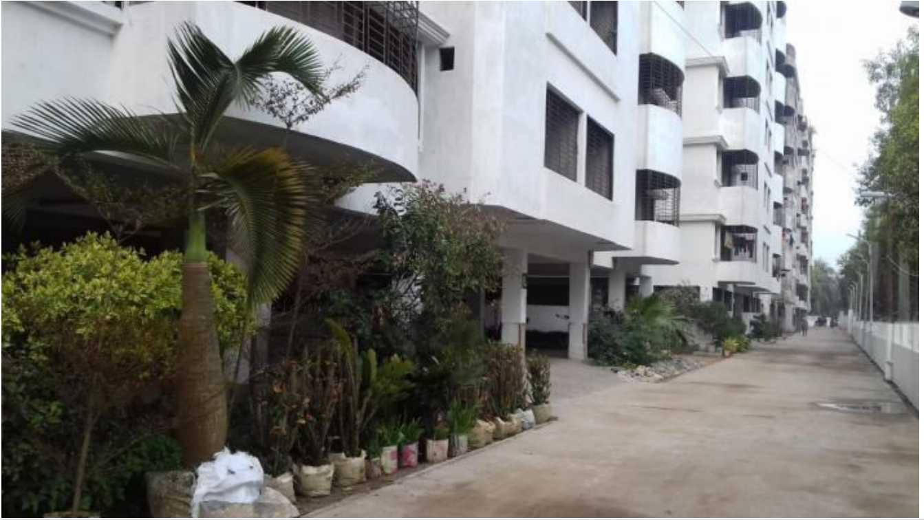
Building- outside plastering
