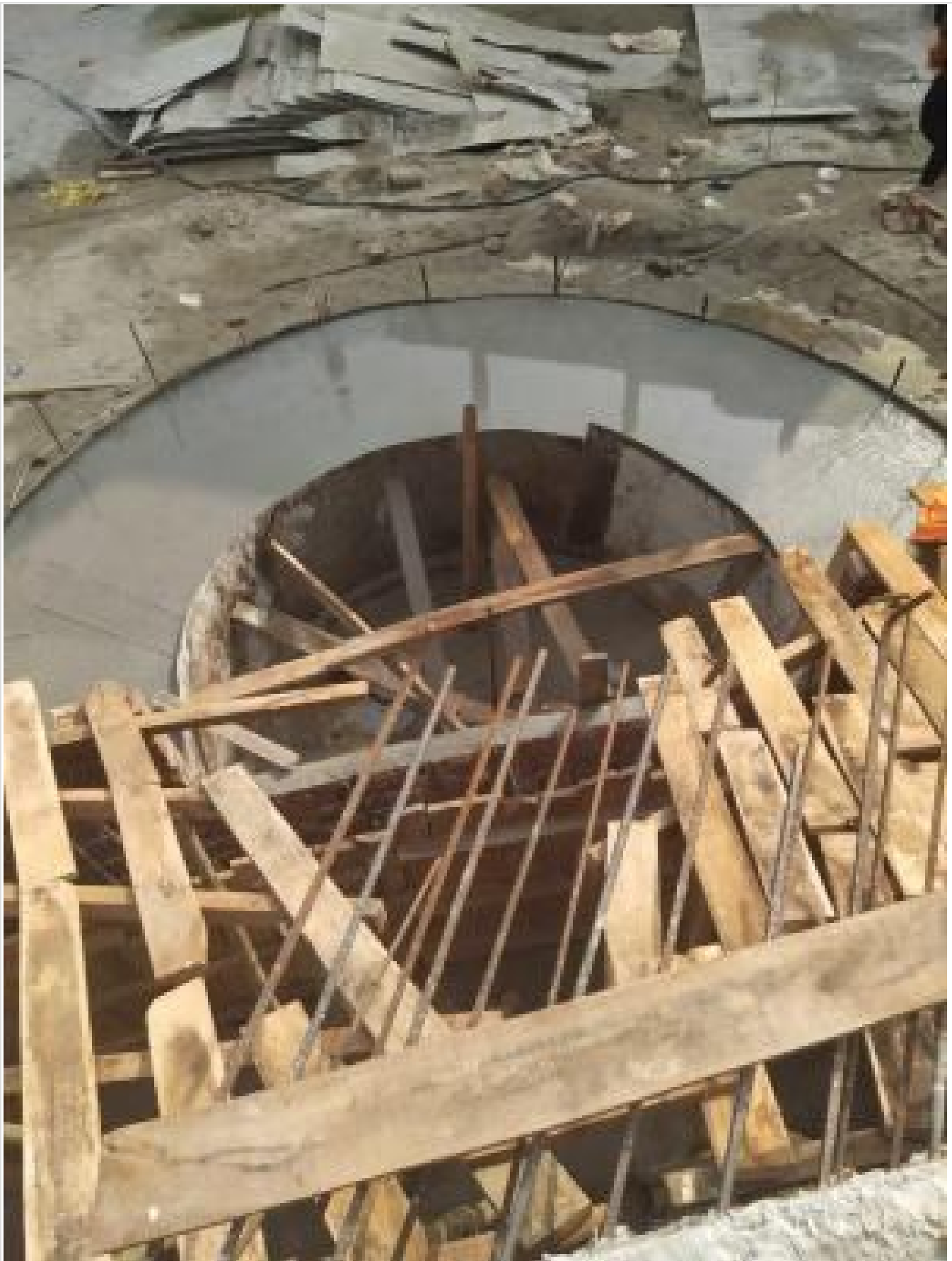
Mosque Ground Floor Stair Concreting
