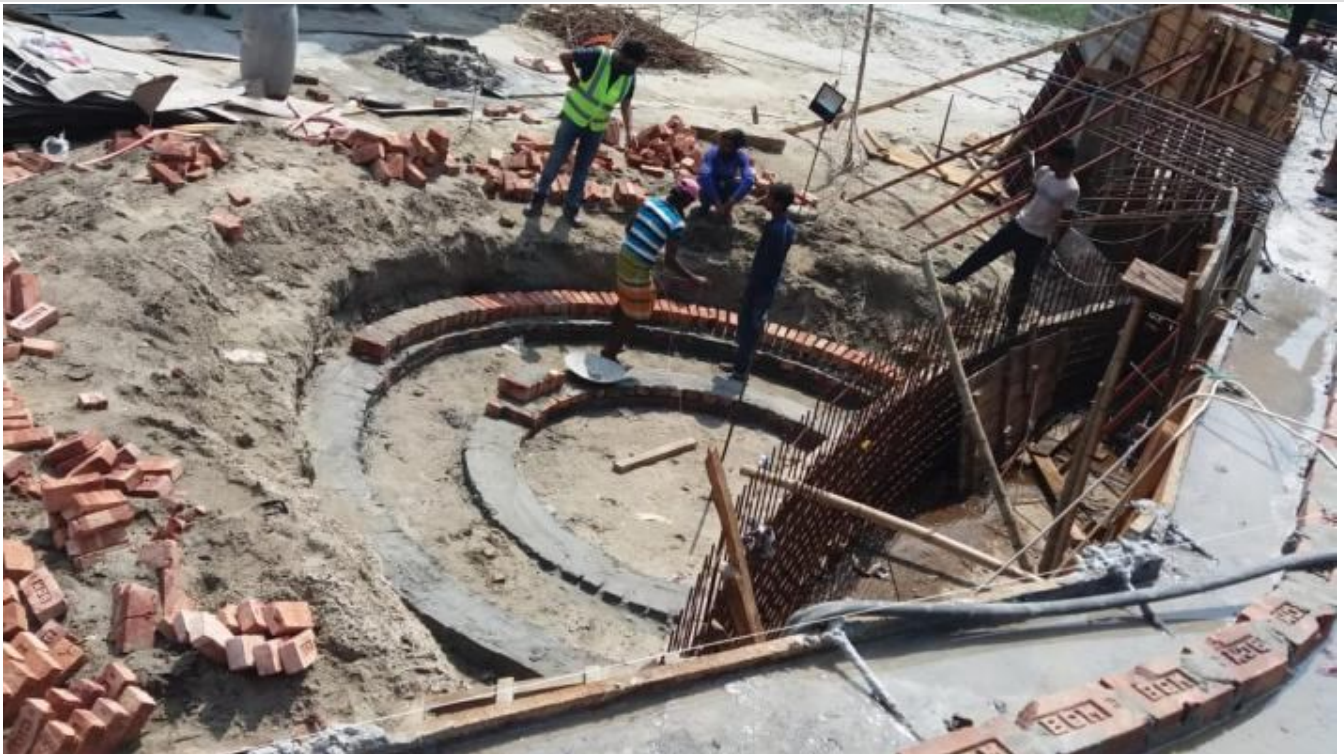
Mosque-GF-Stair Case Foundation Work
